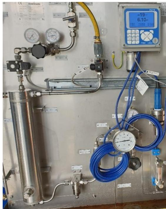
Figure 7. Automated water sampler for measuring DO, pH and ORP in cooled and depressurized brine.
