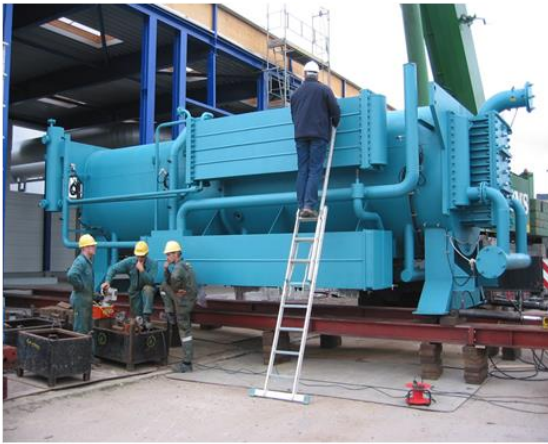
Figur 33: Absorptionsvarmepumpe under installation (Amager)
